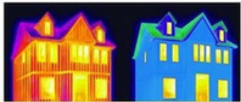
Thermal image of a conventional build.
